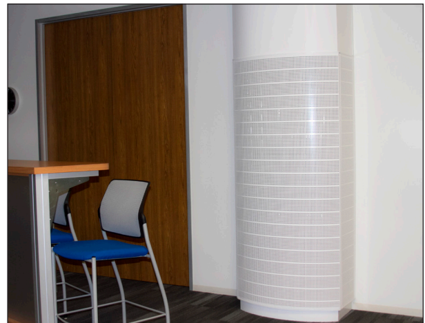
DVBC displacement diffuser installed in a training room with duct cover and mounting base
