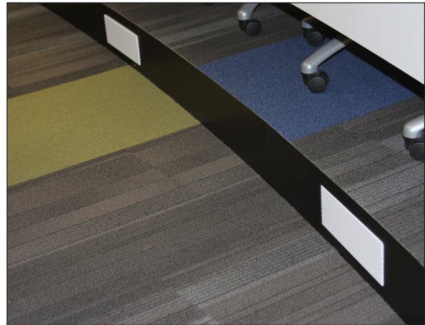
DVR1 units installed in a stair riser
