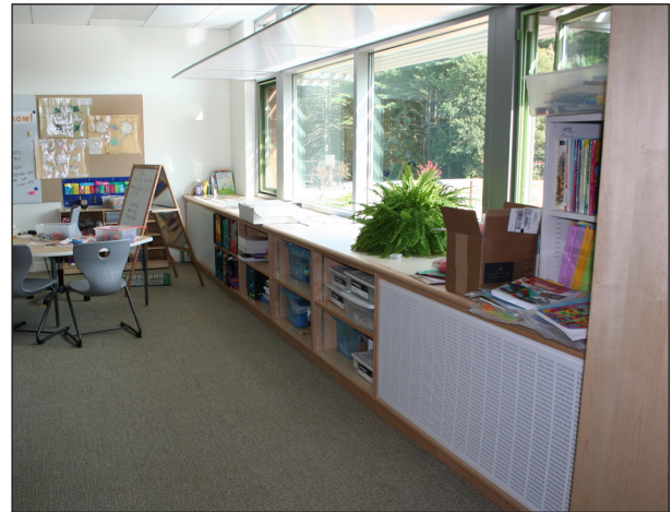
DVIR units installed in the bookshelf of a classroom in an elementary school along the perimeter
