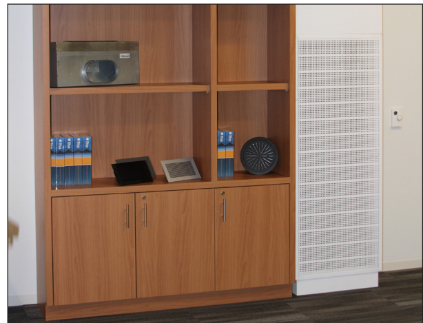
DVR3 unit installed along the wall next to a bookshelf with duct cover and mounting base
